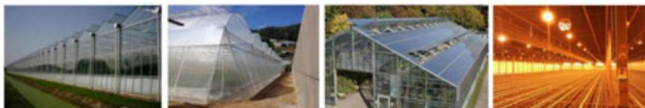
a. A typical multi-span structures of Dutch greenhouse with glass panel for large-scale commercial production
